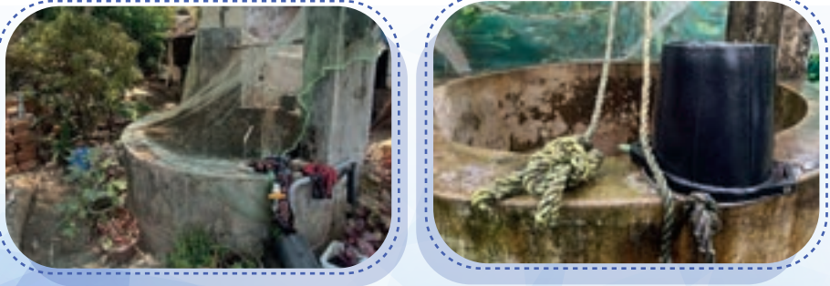
Figure 24. Photographs showing open wells covered with plastic net and coir in Meenchanda Ward, Kozhikode Corporation.
